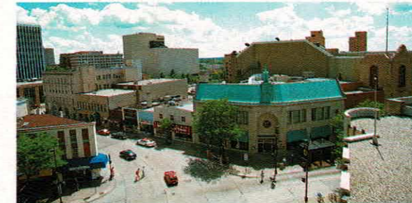
JUNE 2001: Overture Center construction is about to begin.
