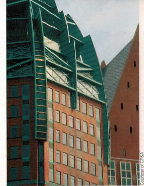
This Cesar Pelli design, a tower in The Hague, Netherlands, extends the city fabric into an area that was bombed during World War II.
