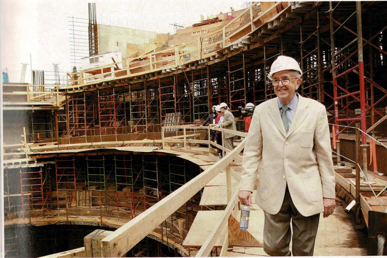
Cesar Pelli tours the Overture Center during construction in 2003: "I have designed a building to feel like Madison."
